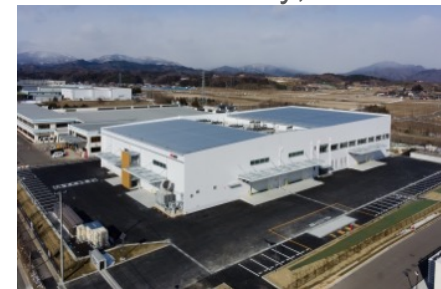
Lab testing: Smart System Research Facility, AIST
