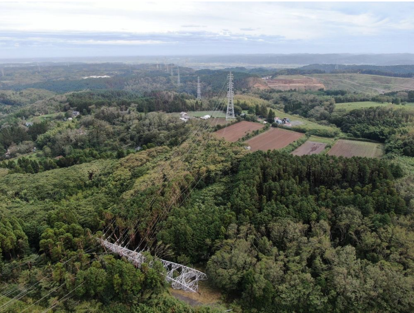
Steel tower collapsed in Chiba, Japan
